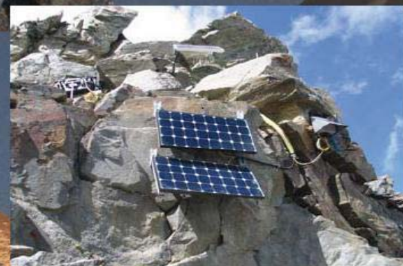
Base station and solar panels on the field site at Matterhorn
